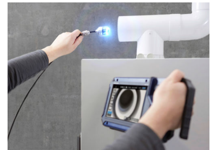
Inspection of flue gas lines from 2": easily negotiates tight bends of 87°.
