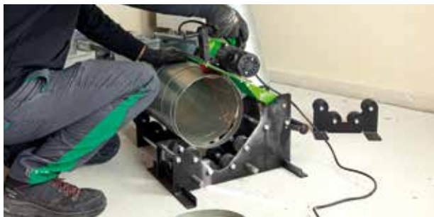
Time-saving cutting of ventilation pipes
